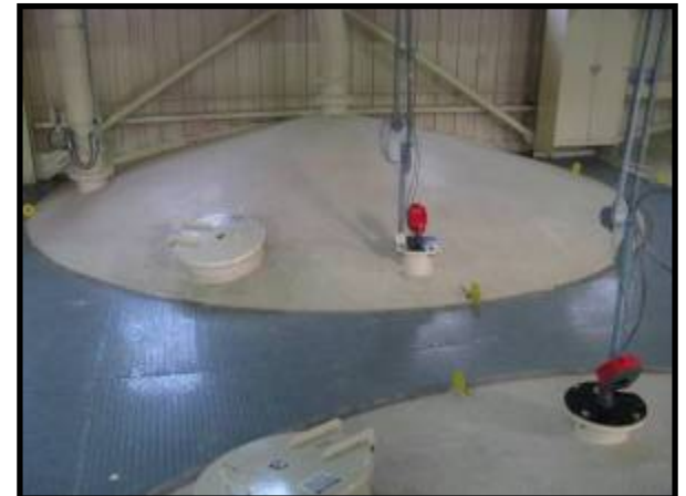
Scanners are installed on 21 silos.
