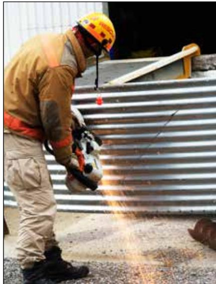
*Method for cutting a “V”-shaped opening into a corrugated steel wall is demonstrated during a 2009 bin rescue workshop at Star of the West Milling Co. in Gera, MI. Photos by Ed Zdrojewski.*
